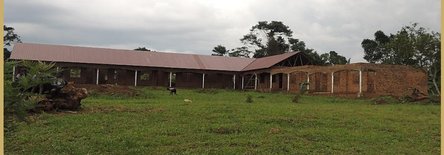
3 rd building under construction with 7 classrooms
