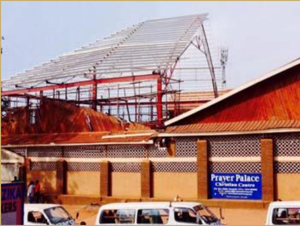
Roof Under Construction
