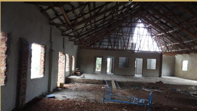
Inside Main Building
