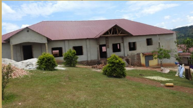
Main Building Under Construction
