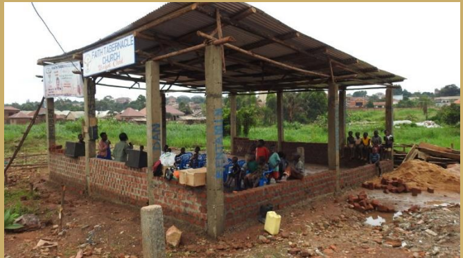
Faith Tabernacle Under Construction
