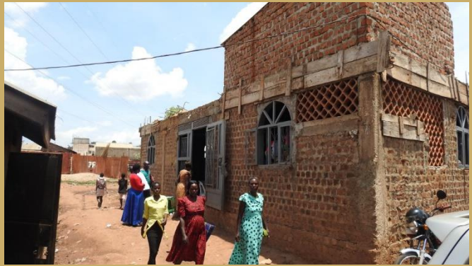
Antioch Church Under Construction
