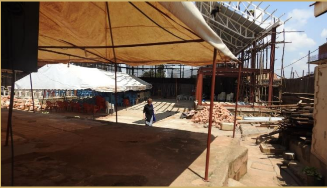
Construction at Prayer Palace
