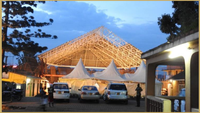
Roof Under Construction
